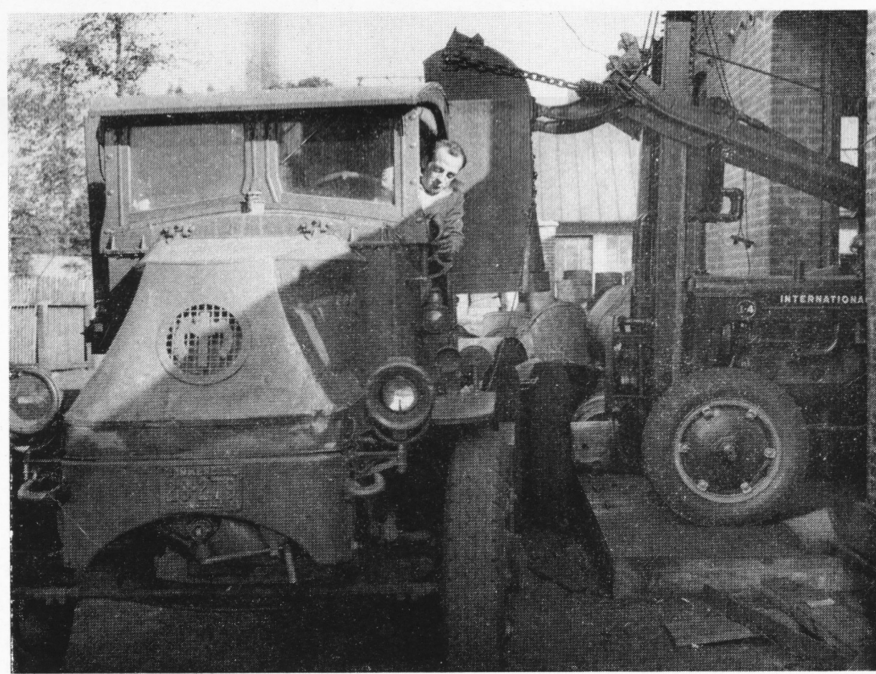
A. Domizio takes a truckload of iron scrap to the railroad freight cars and unloads. When freight cars are loaded they are routed out of Scovill City to metal refineries or other plants which are buyers of scrap material. Shoveling steel, dirty brass, iron brass, etc., all go.
